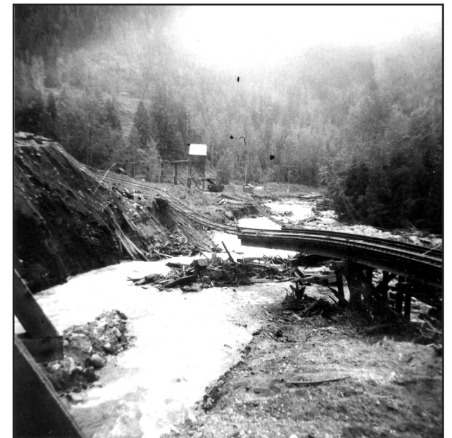
The 1955 flash flood which demolished Sandon also swept away the railway bridge across the creek. Photo: Mary Carne
