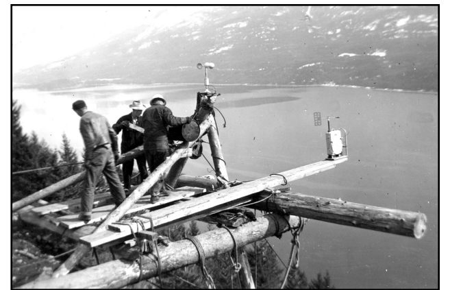
Installing the A-frame and rubbing log at the crest of the 1300' Coffee Creek bluffs in 1952. This low-tech solution protected the power cables as they were being winched up and over the cliff edge to the west towers. Photo: Mary Carne, courtesy of Gray Creek Historical Society
