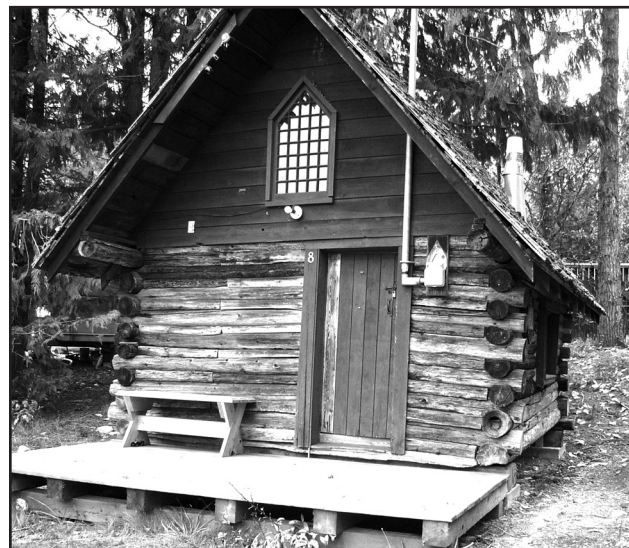
The Redding Cabin, the oldest building in Gray Creek, was built of fire - killed cedar in the 1890s. The cabin is now located next to Gray Creek Hall and is being rehabilitated for community use. Visit the cabin and interpretive sign on the Hall property, or you can read all about it in the Gray Creek Tour Guide brochure - free at local stores.
