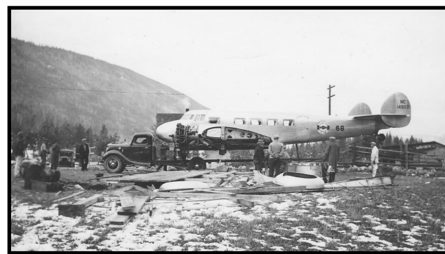
Framing removed; plane secured on trailer
