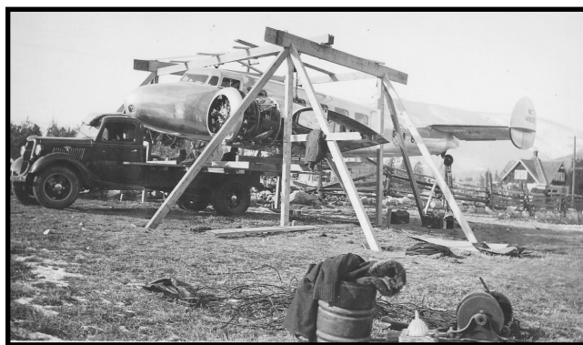
Flatbed trailer backed in under fuselage; wings, propellers and engine cowlings removed
