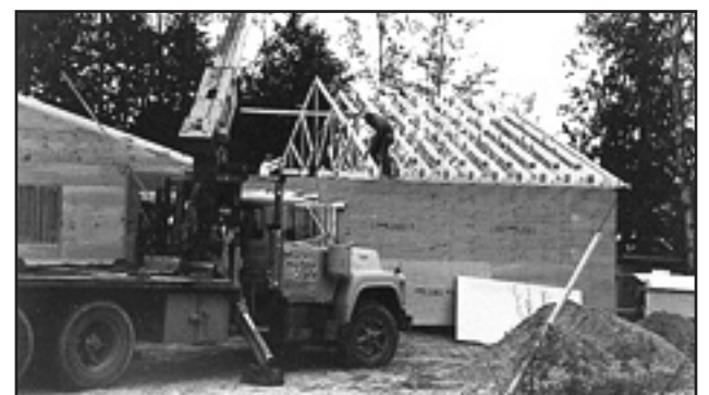
Bluebell Manor being built in 1987
