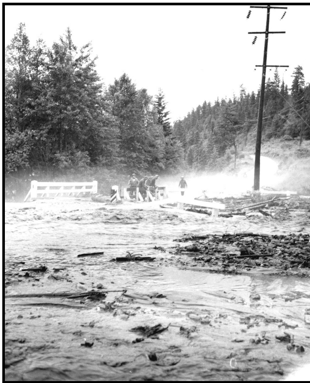
Lockhart Creek floods the highway, but the new bridge holds up - luckily for this road crew. June 1955. Photo: GCHS, courtesy of Hephher family
