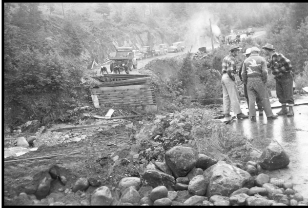
Bridge washout at Sanca Creek, June 1955. Photo: GCHS, courtesy Mary Carne
