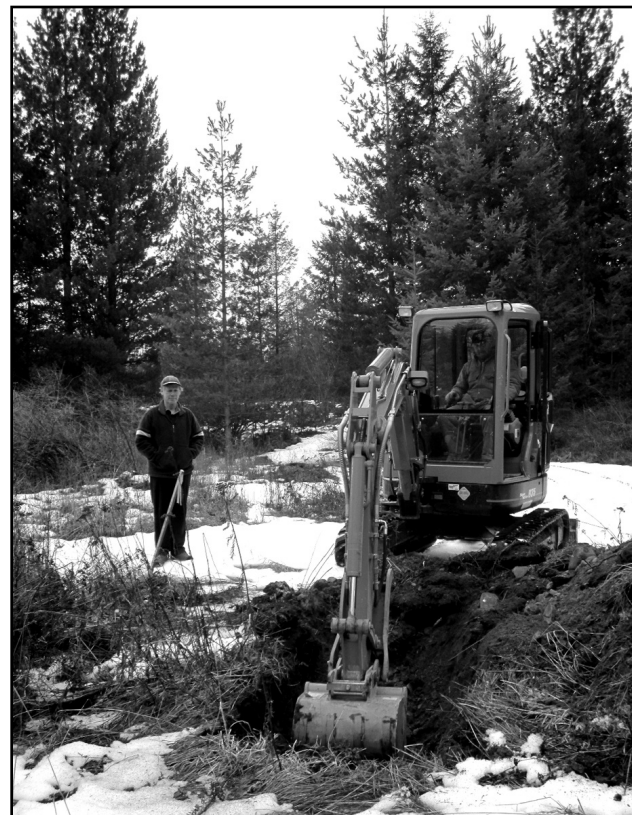
Glen Kinder looks on as Dave Hough of Steel Wheels digs observation pits to ascertain septic capability on the land KLEECA is developing for senior’s housing in Crawford Bay
