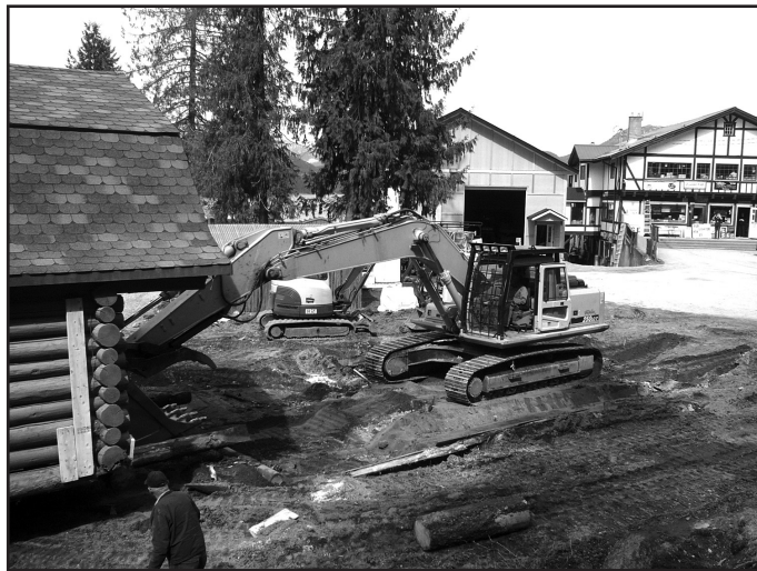
Ray Besanger uses the bucket of his machine to push the lodge back on log rollers set under the building. Photo: Tom Lymbery
