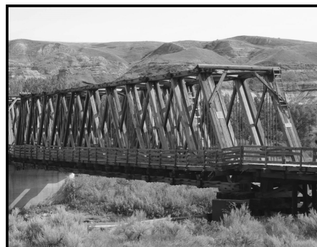
Example of an old Howe truss bridge, this one at East Coulee, Alberta. Photo (detail): Facebook
